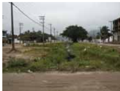
PGR28PON51FOT02 - Canal do Praião com as vias marginais
