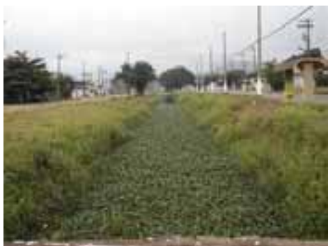
PGR28PON50FOT01 - Canal do Praião com as vias marginais
