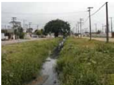
PGR28PON51FOT01 - Canal do Praião com as vias marginais
